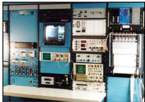
Figure 18 FESI Data Acquisition Equipment Room
