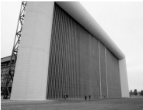
Figure 22.6 Inlet for the NASA Ames wind tunnel being used for testing wind turbine rotor and blade configurations
