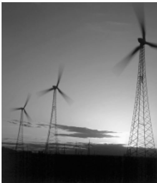
Figure 22.1 This 193-MW wind power plant at Storm Lake, Iowa uses Zond Energy Systems 750-kW turbines
