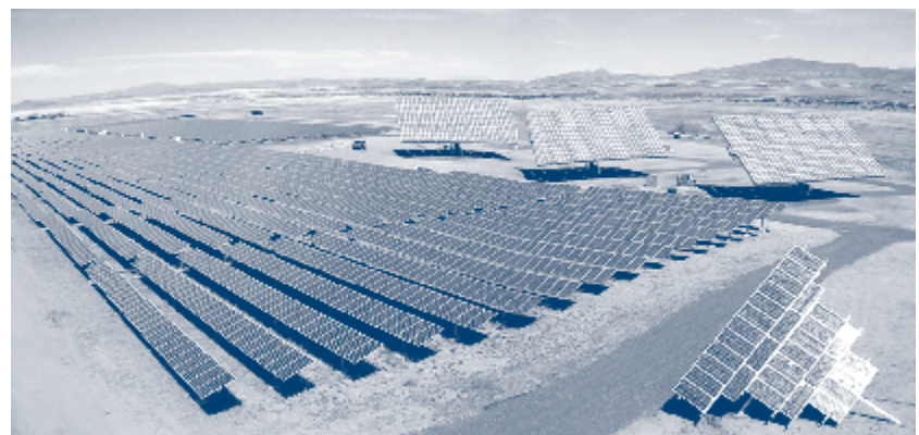
Figure 5. PV systems at the Arizona Public Service facility in Prescott, AZ, use a combination of technologies. The systems in the foreground are single-axis-tracking, flat-plate silicon systems. Shown in the upper right are three large (35-kW) Amonix CPV systems. The data in Figure 4 were obtained from systems such as these.
