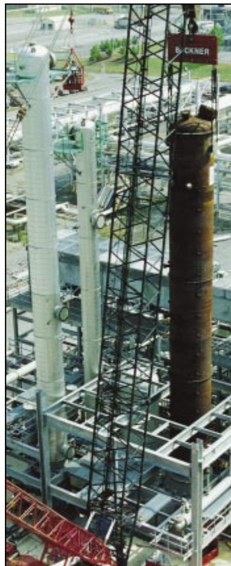
Erection of the reactor vessel at the LPMEOH™ Demonstration Unit.
