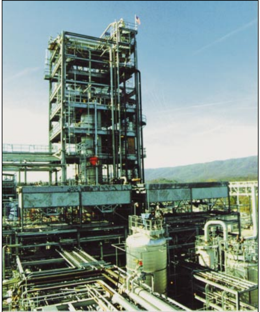
LPMEOH™ Demonstration Unit.
