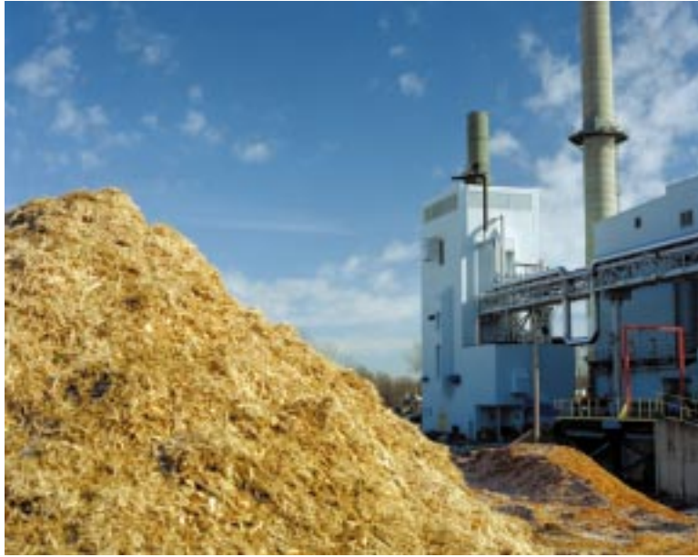
The Battelle gasifier in Burlington, Vermont, provides a clean gas fuel for modern power systems that can achieve efficiencies double those of today's biopower industry.
