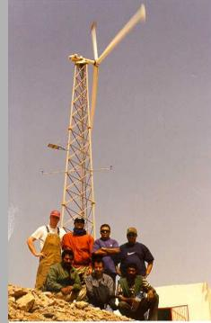
Using one AOC 15/50 (50Hz), two 50 kW diesel generators, and 1.5 miles of 2400 volt overhead power line, the system powers a 12 ton per day ice maker, irrigation pumping, crop processing, and lighting and refrigeration for the housing complex.
